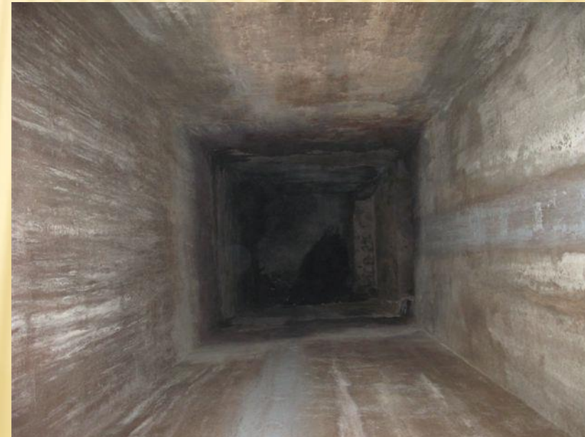
Shotcrete Restoration Permacast MS 10000 + ConShield
