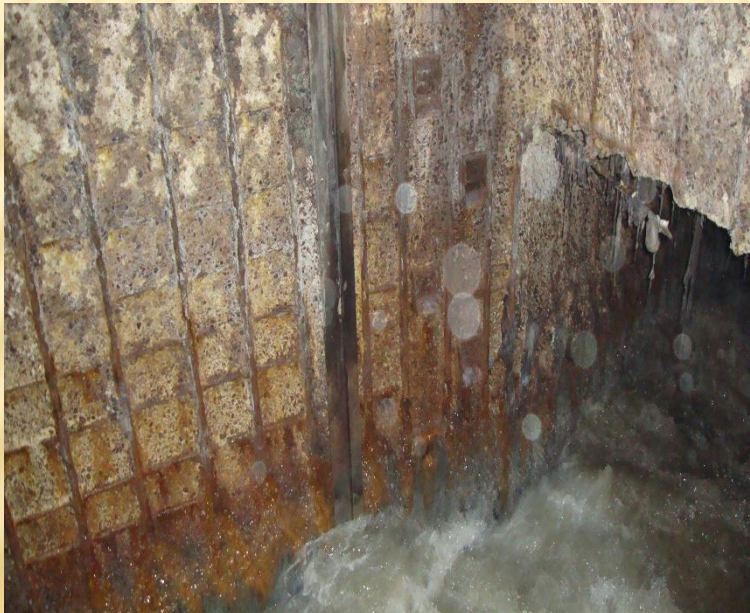
MIC Damage – 5" Concrete Loss After only (3) years of Service
