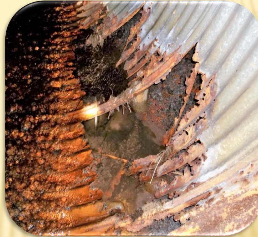
Hydrated Iron Oxides (Rust)
